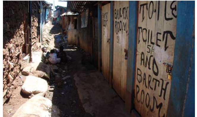
Unregulated, informal sanitation service providers do not comply with human right standards, Mathare, Nairobi, Kenya © Daniel Nordmann
