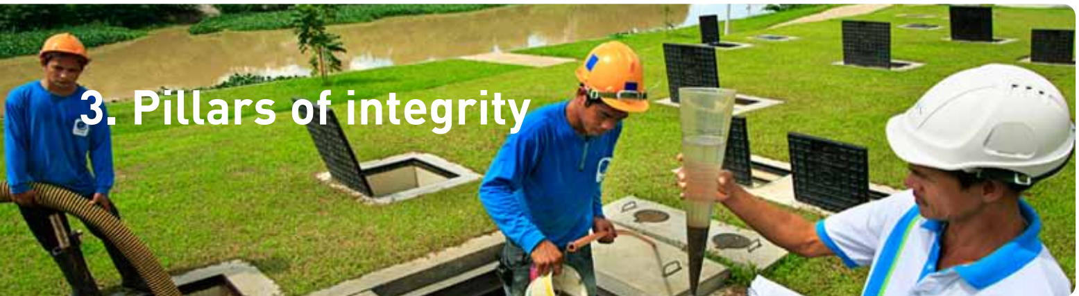
Water treatment: Part of an effort to rehabilitate the Pasig river, a sewage treatment plant was constructed in Marikina city (Philippines) where waste water collected from residential and commercial establishment is treated and recycled. © Danilo Victoriano, finalist WIN photo competition 2011
